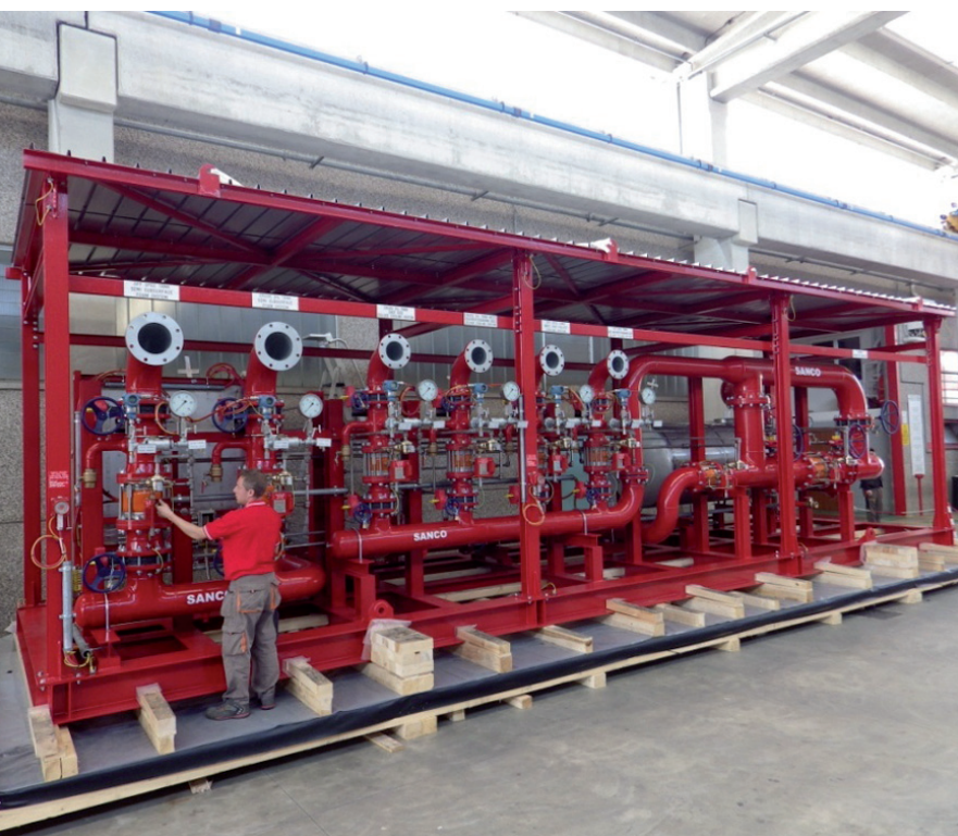
Fig. 2 - Deluge valves on skid
