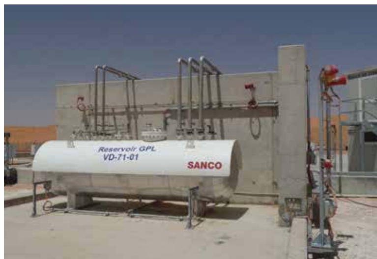
Fig. 7 - Fire training ground LPG vessel
