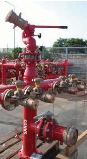
Fig. 3 – Kuwait project: fire monitor on hydrant
