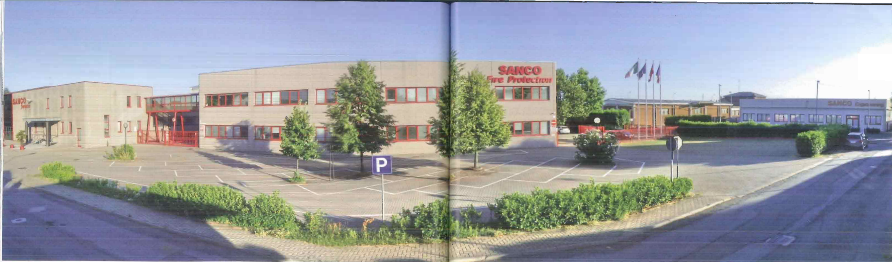
Fig. 1 –Sanco's headquarters in Galliate, Italy
