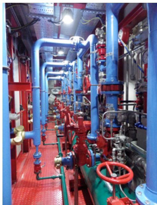
Internal view of one deluge valve container for Russia
