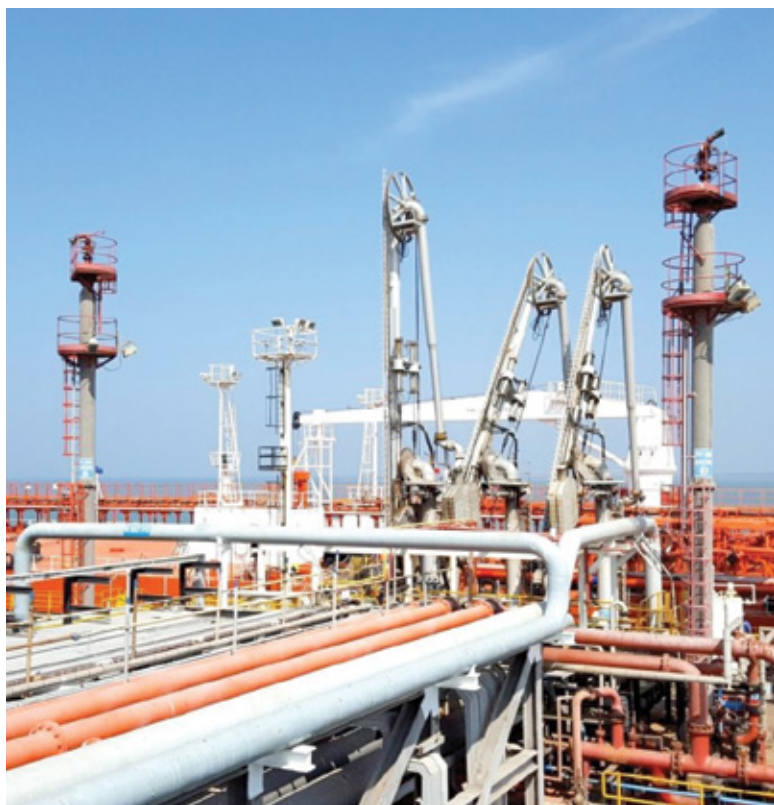
Remote controlled monitors on towers
